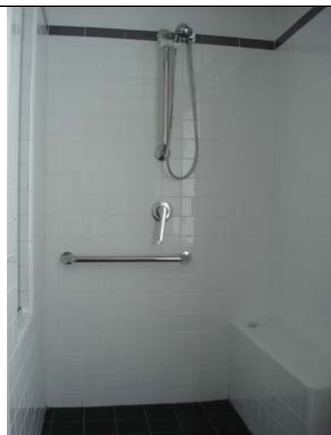
Photo: Shower area with tiles seat.
