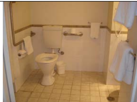
Photo: Toilet, grab rails and circulation space.
