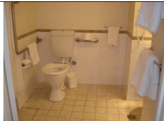
Photo: Toilet, grab rails and circulation space.
