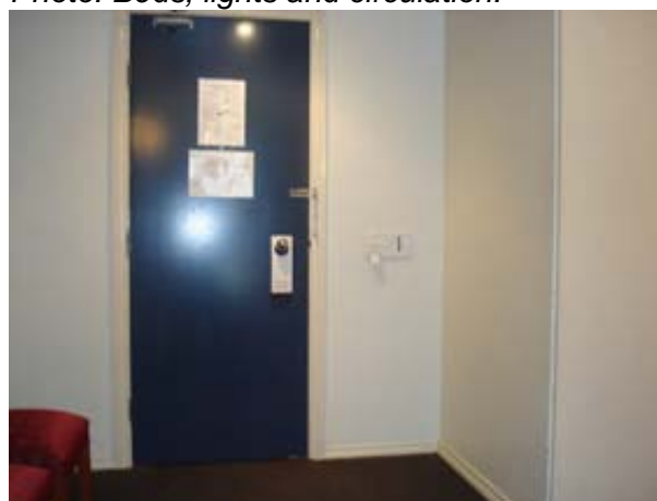
Photo: Showing entry, door knob, closer and latchside space.
