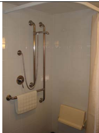
Photo: Roll- in shower, lever tap and grab rail. Note the small shower seat.
