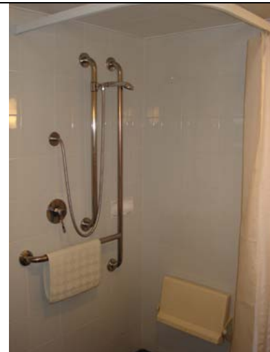
Photo: Roll- in shower, lever tap and grab rail. Note the small shower seat.
