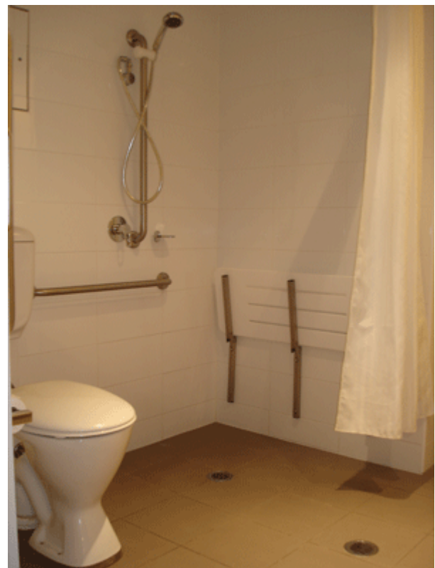
Photo: Toilet and grab rails. Roll-in shower, grab rail
