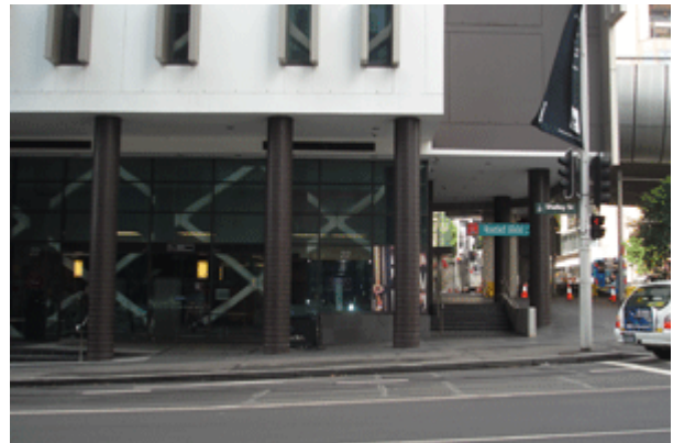
Photo: Entry from Shelley St.
