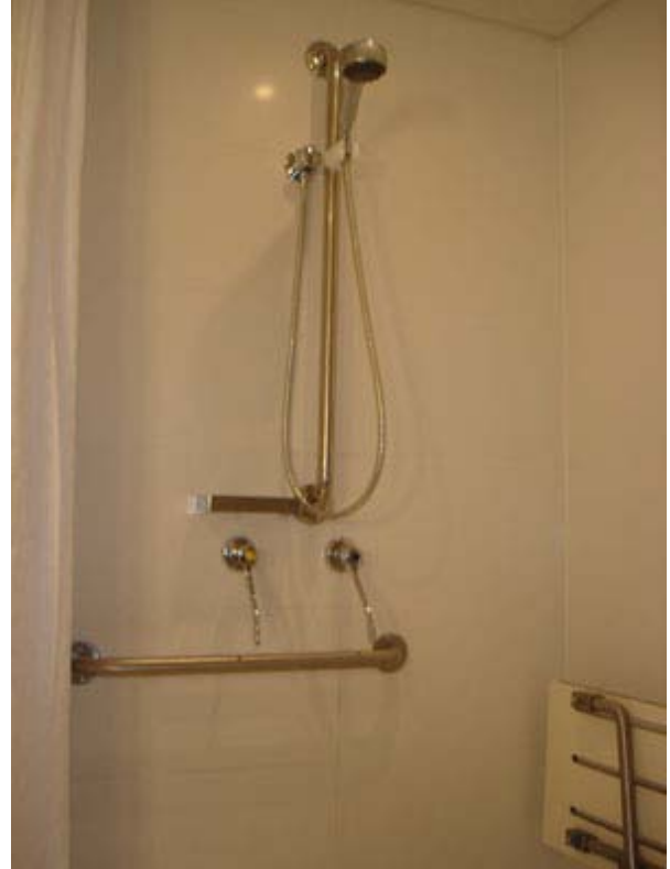
Photo: Shower, grab rail and shower seat
