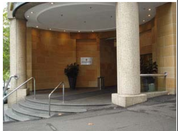
Photo: Entry from Cnr Bridge and Phillip Sts.
