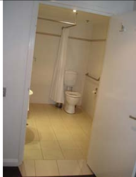
Photo: Bathroom entry, graded tiles up and toilet/grab rail.
