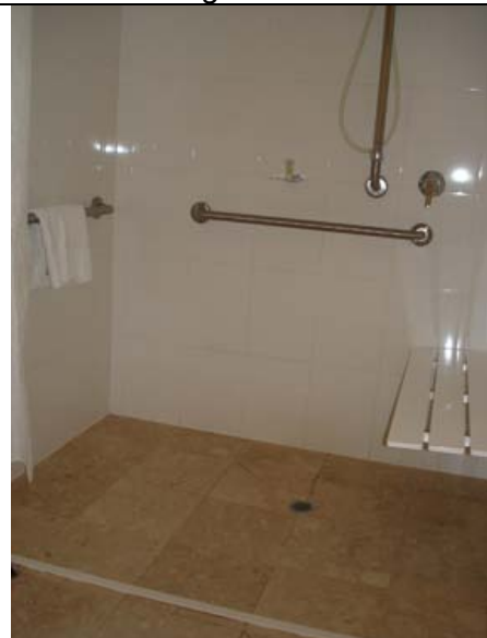
Photo: Shower area with plastic strip on the floor and fold down shower seat.
