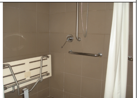
Photo: Shower area with plastic strip on the floor and fold down shower seat.
