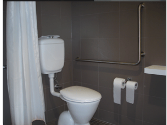
Photo: Toilet, grab rails and shower.
