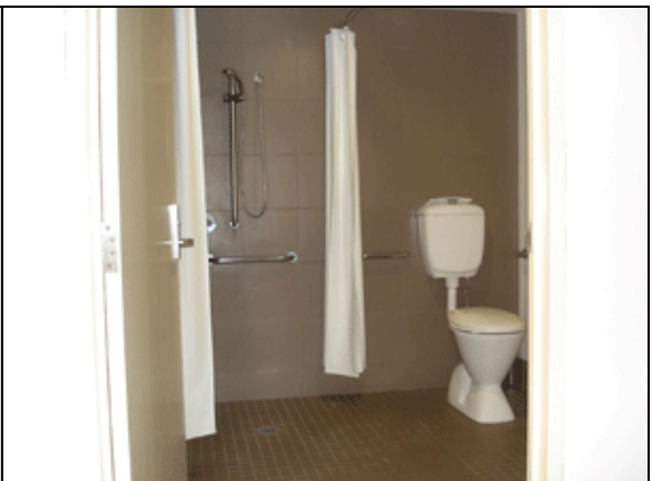
Photo: Toilet, grab rails and shower.
