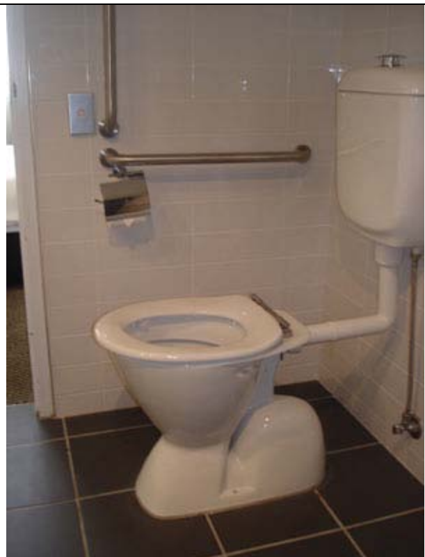
Photo: Toilet and grab rails.
