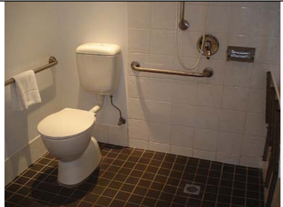
Photo: Toilet, grabrail and shower area.
