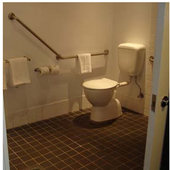
Photo: Through sliding door showing toilet & grab rail.
